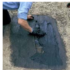
PRIOR TO REPAIRS
