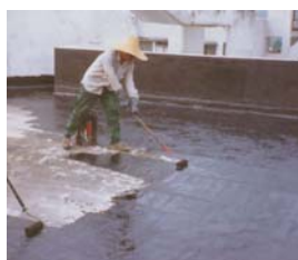
PRIOR TO COATING
