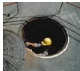
SUBGRADE UTILITY USE
