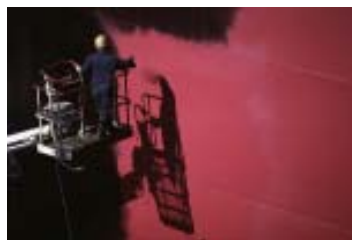
Outdoor metal tanks
